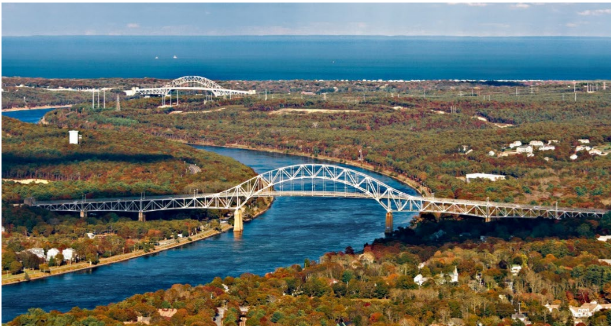
Figure ES-7 – Looking Northeast at the Bourne (foreground) and Sagamore Highway Bridges
